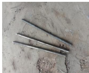
Figure 11. Fabrication of the reinforcing steel length
