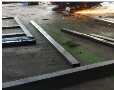
Figure 5. Fabrication of the lower frame inclination
