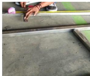
Figure 4. Fabrication of the lower frame
