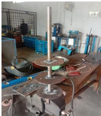
Figure 15. Fabrication of the hammer frame
